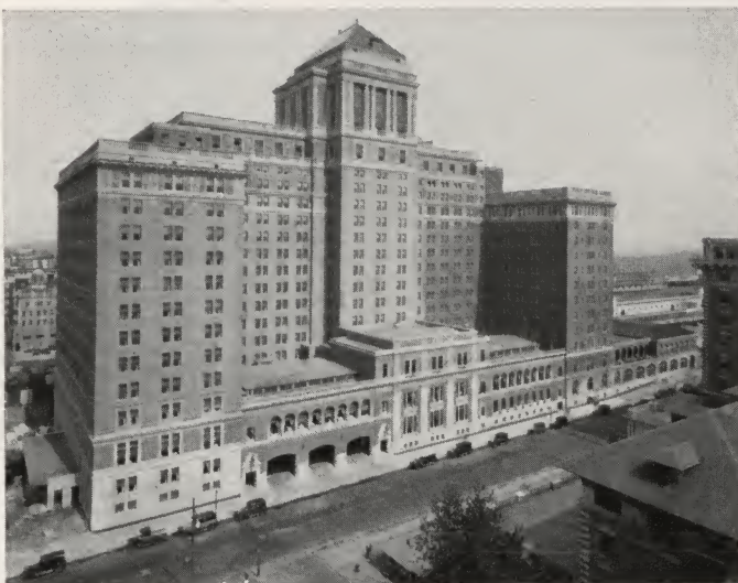
Left center —Approximately 500,000 concrete masonry units were used as backup in the popular Haddon Hall at Atlantic City. A great many of the partitions are also firesafe concrete masonry. Rankin and Kellogg, architects. Turner Construction Co., contractor.
